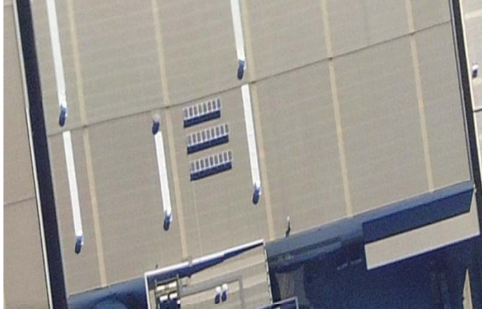
CSR-NSW Factory (installed)
